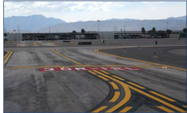
Holding Position Marking, Enhanced Taxiway Centerline, and In-Pavement RGLs
