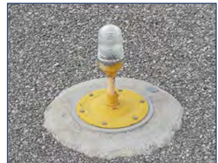
Medium Intensity Runway Light (MIRL) Fixture
